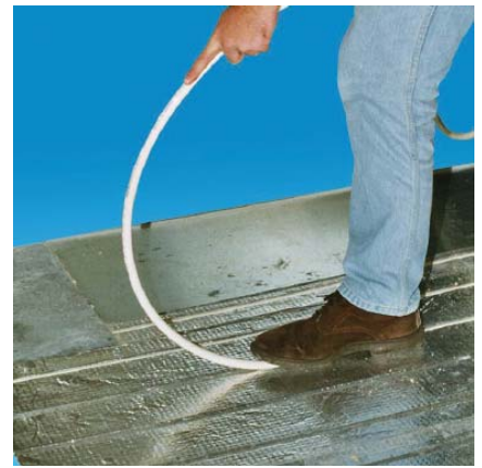
Pressing down of the heating pipes
