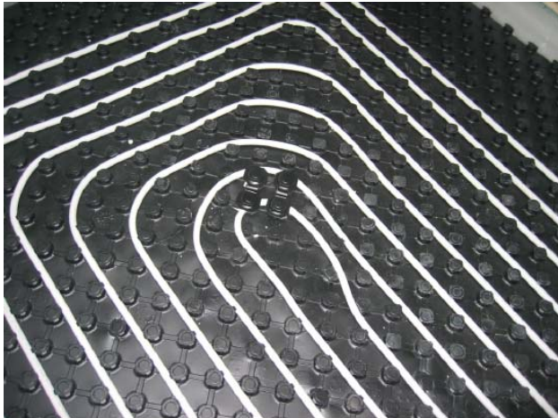
Heating for floors with nap plate system components
