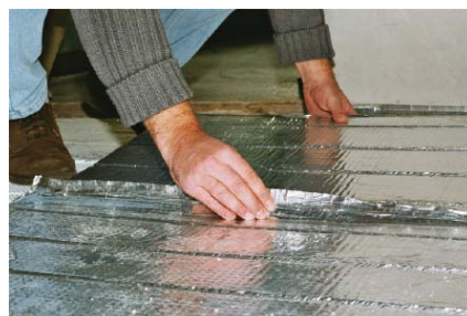
Laying of multi-clamp plates and overlapping of the sticking foil
