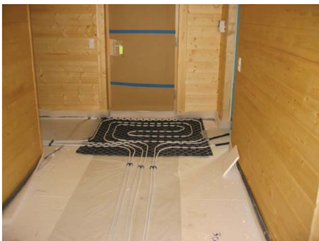
Distributed pipe and plate system for heating in the hallway
