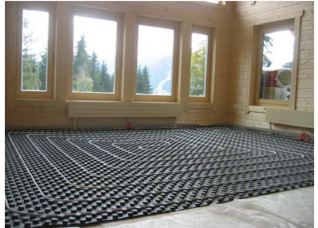
Heating for floor with nap plate system components
