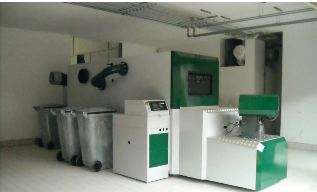
Biomassekessel, Feriendorf Vila Vita Pannonia, Parndorf
