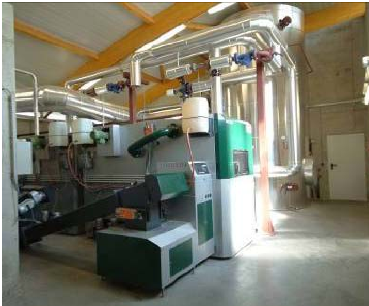
Kesselraum / Boiler room:
