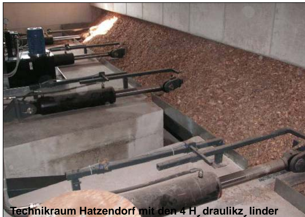
Schema: 2-reihige Schubstange Scheme: 2-row walking floor
