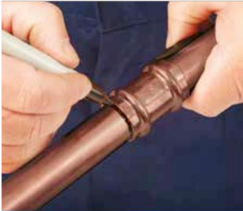
4. Assemble and mark the insertion depth
