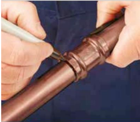
4. Assemble and mark the insertion depth
