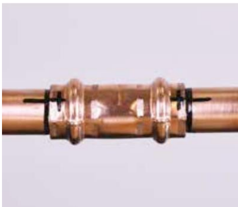
6. Mark the completed joint
