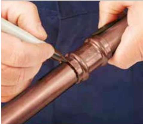
4. Assemble and mark the insertion depth
