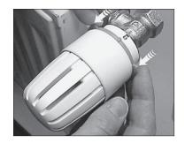
The locking sleeve ③ is unlocked and can be slid towards the locking nut. When this is done, the setting marks of the handwheel become visible. The unlocking tool can be removed.
