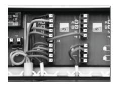
It is possible to assign more than two actuators to one thermostat by a wire strap.
