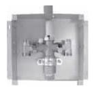
**4.** Attach the thermostat element on the wall, in consideration of the available capillary tube length, so that the arrow on the base plate points upwards. Depending on the model, the thermostat element is mounted on the wall or in a flush-mounted socket.
