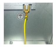
During servicing work the protective earth connection for the front door can be released. It is essential to re-establish this connection after servicing work.
