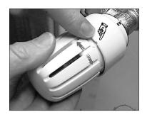
Then, without tools, slide the locking sleeve towards the handwheel until the hand wheel scale is covered and the sleeve clicks into position.
