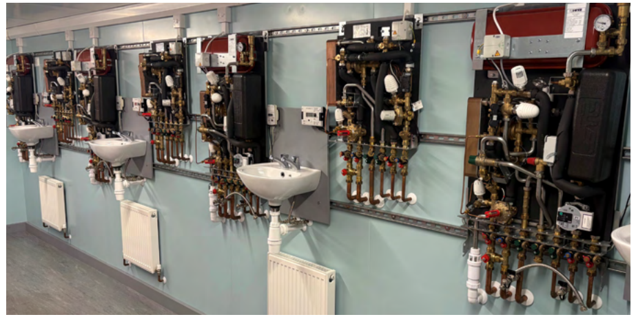
Training centre on the premises of HERZ Valves UK in Peterborough.
