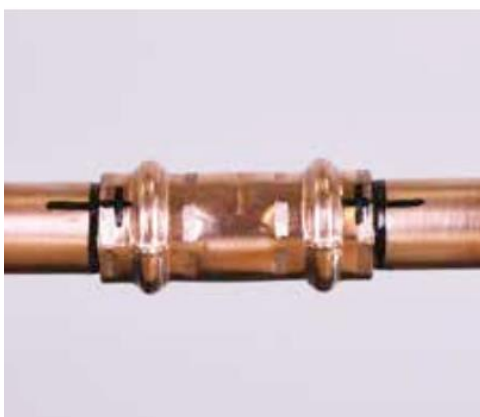
6. Mark the completed joint
