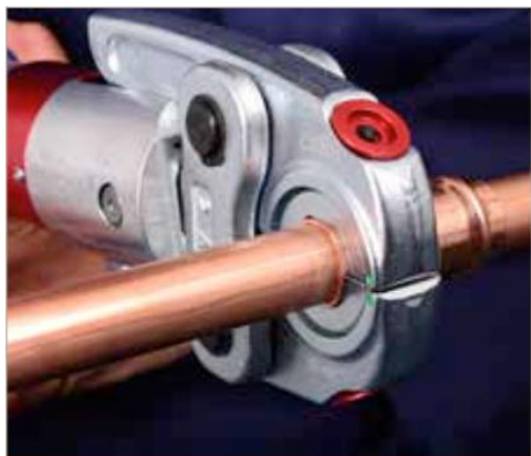
5. Complete the joint with the press tool
