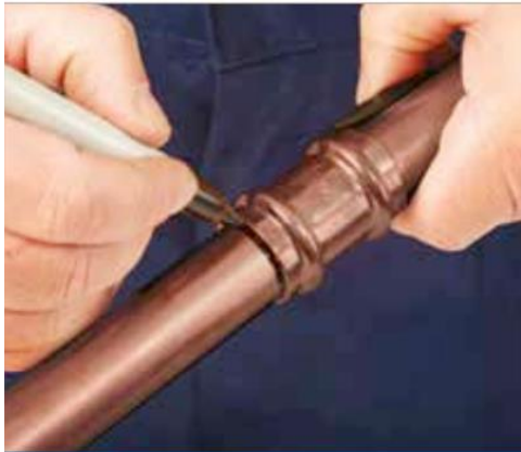
4. Assemble and mark the insertion depth
