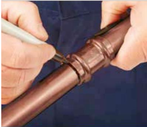
4. Assemble and mark the insertion depth
